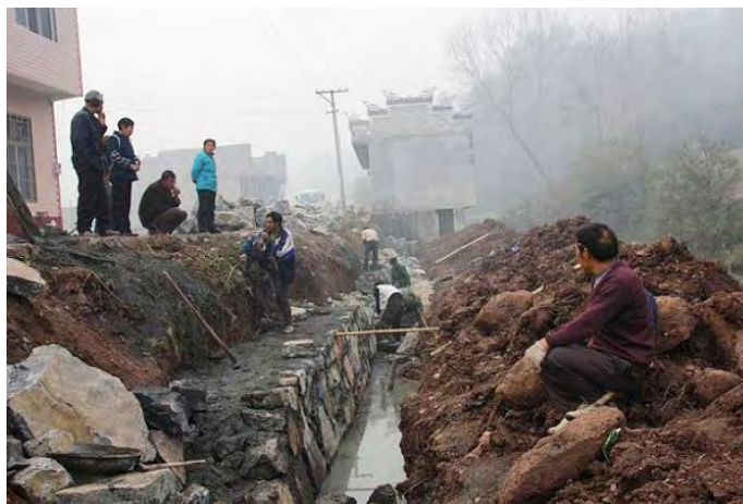
Villagers supported by the Federation's community based disaster preparedness programme worked on reinforcing a river embankment to reduce their risks in future floods. January 2009. Hubei branch of the RCSC.
