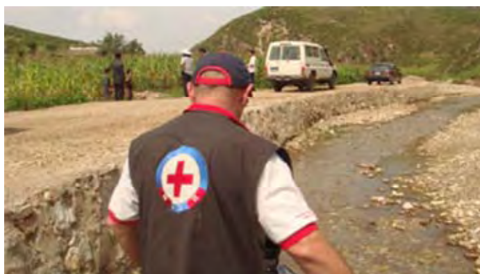
River bank reinforcement under construction by community volunteers, Jongchuk Farm, Songchon county, South Pyongan province in September 2009. Photo: International Federation.
