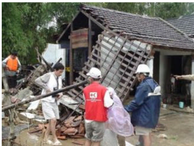
A collapsed house in Hue.
