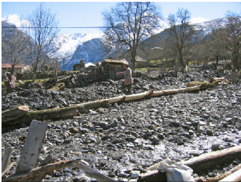
Land of debris: the aftermath of the disaster has been devastating for many villages.
