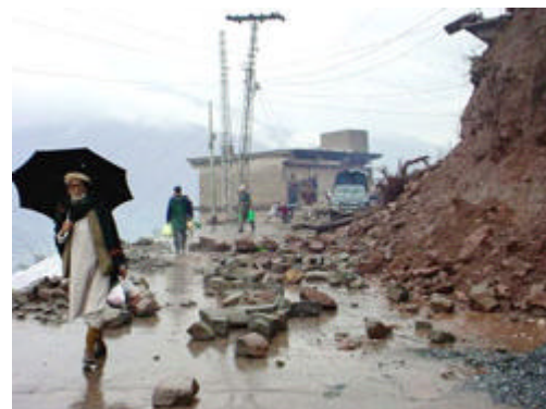
Men walk along a road damaged by a landslide in Muzaffarabad (REUTERS/Amiruddin Mughal/courtesy www.Alertnet.org)
