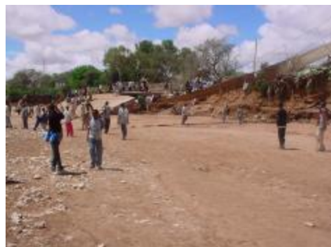
Residents of Hargiesa assess the damage caused by floods to road infrastructure.
