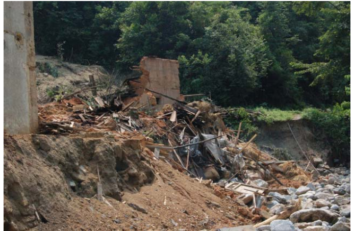
Mudslides triggered by floods have destroyed homes and property in Fujian, Hunan, Guangdong and Zhangzhou provinces
