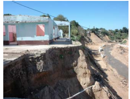
View of the Tartagal River, homes partially destroyed in its banks.
