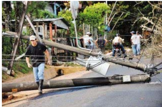
The earthquake damaged electric poles which are blocking roads in an affected area. Source: La Nacion.
