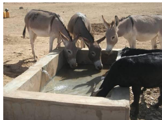
A concrete basin constructed for the watering of livestock in the Brakna region - Photo: MRCS/IFRC
