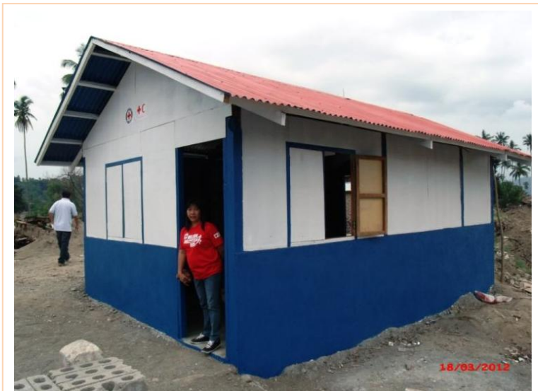
One of the model houses constructed in Iligan City. PRC has started to deliver transitional shelter materials for affected families to rebuild. Photo: Mollie Godinez/PRC
