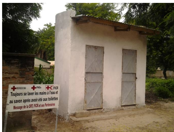
One of the twenty blocks of two latrines built in Kelo, Lai, Bere and Mongo. Some of the latrines are waiting to be handed over to the communities. Photos RCC.
