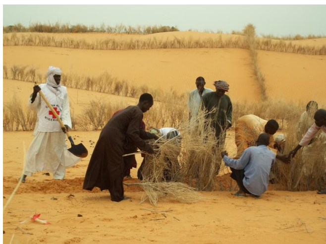
Soil rehabilitation and dune fixing during the Cash-for-work activities in Diffa region: Photo/ RCSN/IFRC Chaibou Kwaini
