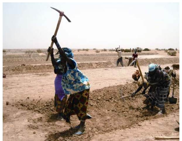
RCSN cash for work activities: Making benches for land recovery in Tillabéry region of Niger (photo Tidjani).
