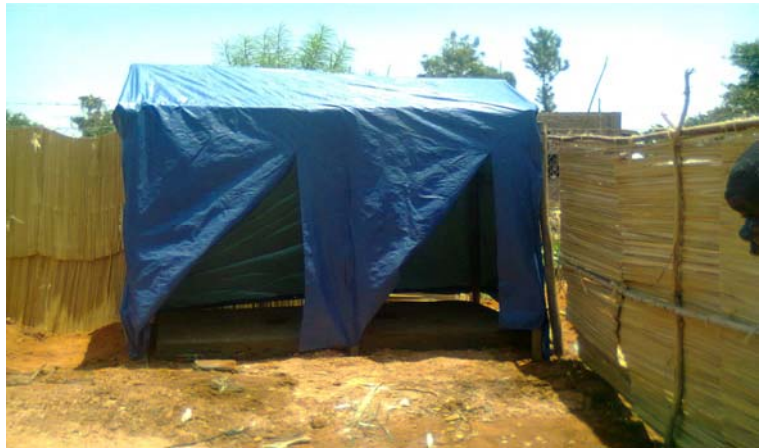
Two-stance emergency latrines constructed to promote safe disposal of human wastes in Namtala – Mbale district: Photo URCS
