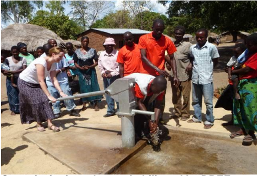
Commissioning a bore rehabilitated by DREF funds in Mangochi: Photo MRCS
