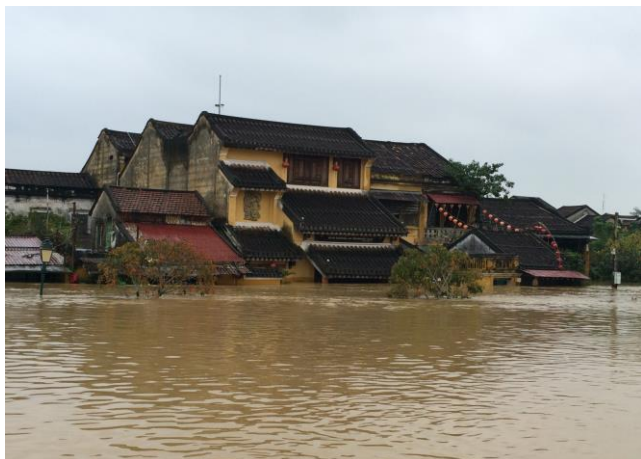
Hoi An city, Quang Nam is under the water. Photo by VNRC Quang Nam Chapter
