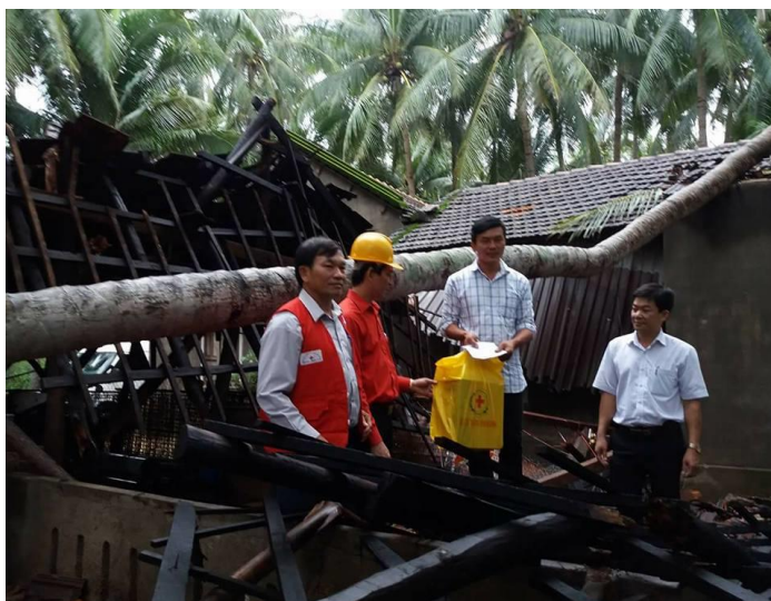
VNRC Binh Dinh Chapter visited and distributed relief and cash to a household whose house was collapsed in Hoai An, Binh Dinh. Photo by VNRC Binh Dinh
