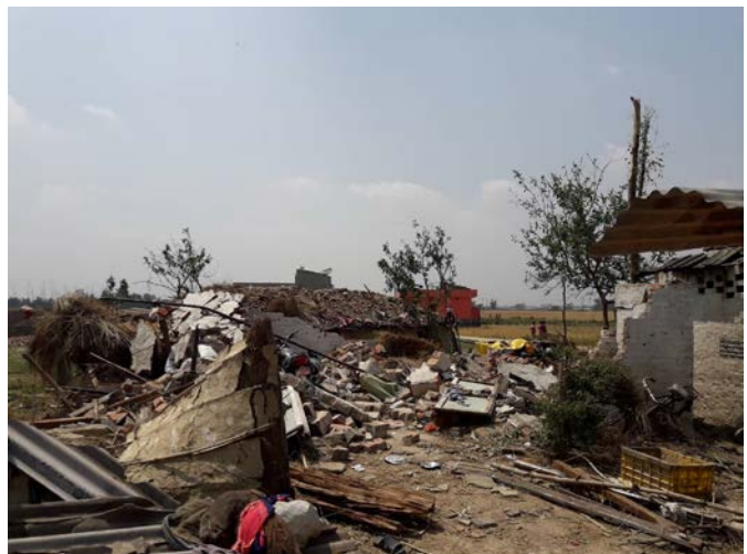
Damage caused by the windstorm in Parsa District. (Photo: NRCS)
