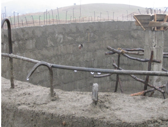
Water storage tank under construction in Samchon County, South Hwanghae Province
