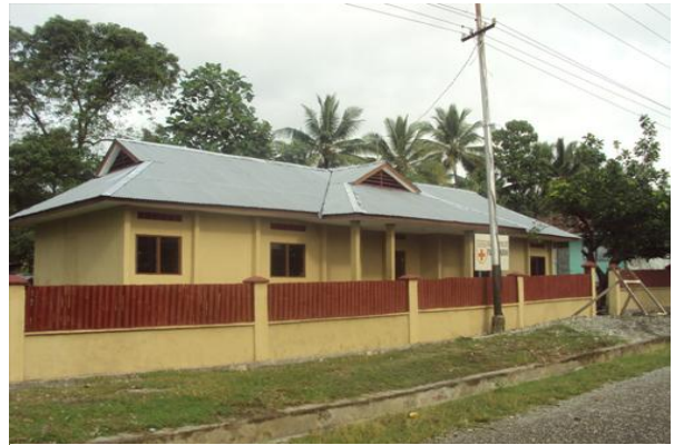
The renovated Manufahi branch building was inaugurated in May. Photo: CVTL
