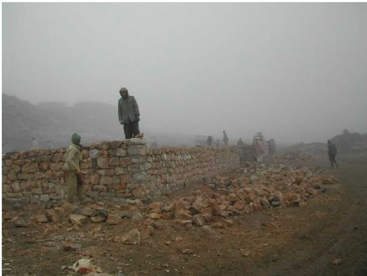
The construction of the schools in Nahrin.
