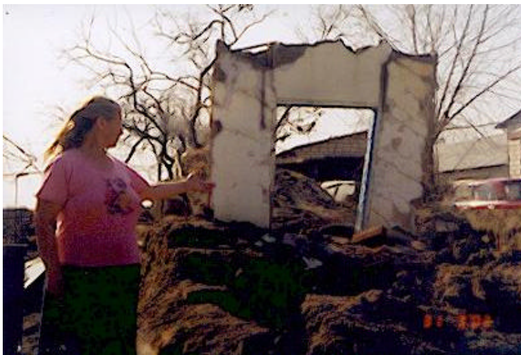
Aftermath: a woman surveys the ruins of her home destroyed by floods.
