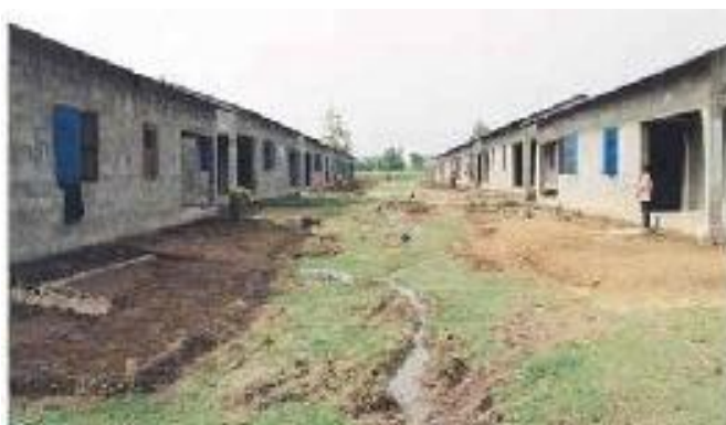
Some of the 225 houses constructed as part of the project
