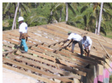
Figure 3 School roof repairs in Cakadrove district.
