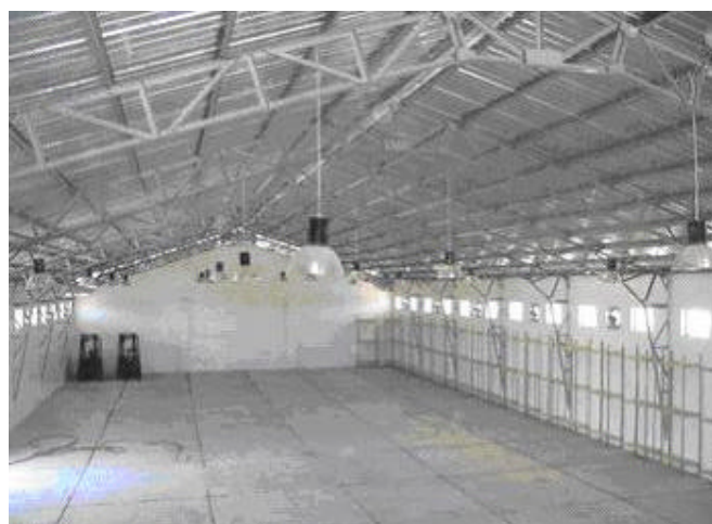
The construction of the Salah-al Din warehouse is completed with bilateral support from donors
