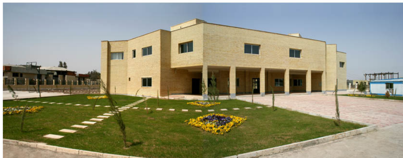
Special Schools for Disabled Children Engineer Mohammed Taheri Hanjani / Primary School
