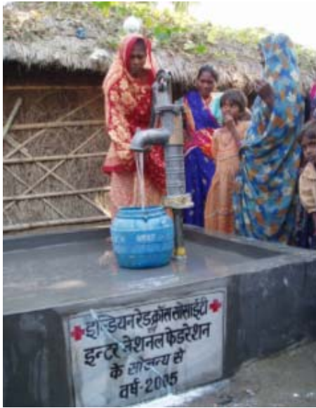
Raised tube wells such as this one in Bihar are proven reliable sources of clean water in times of flood
