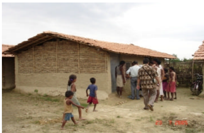
A family inspects one of the 1800 rebuilt/repared houses provided by the Nepal Red Cross
