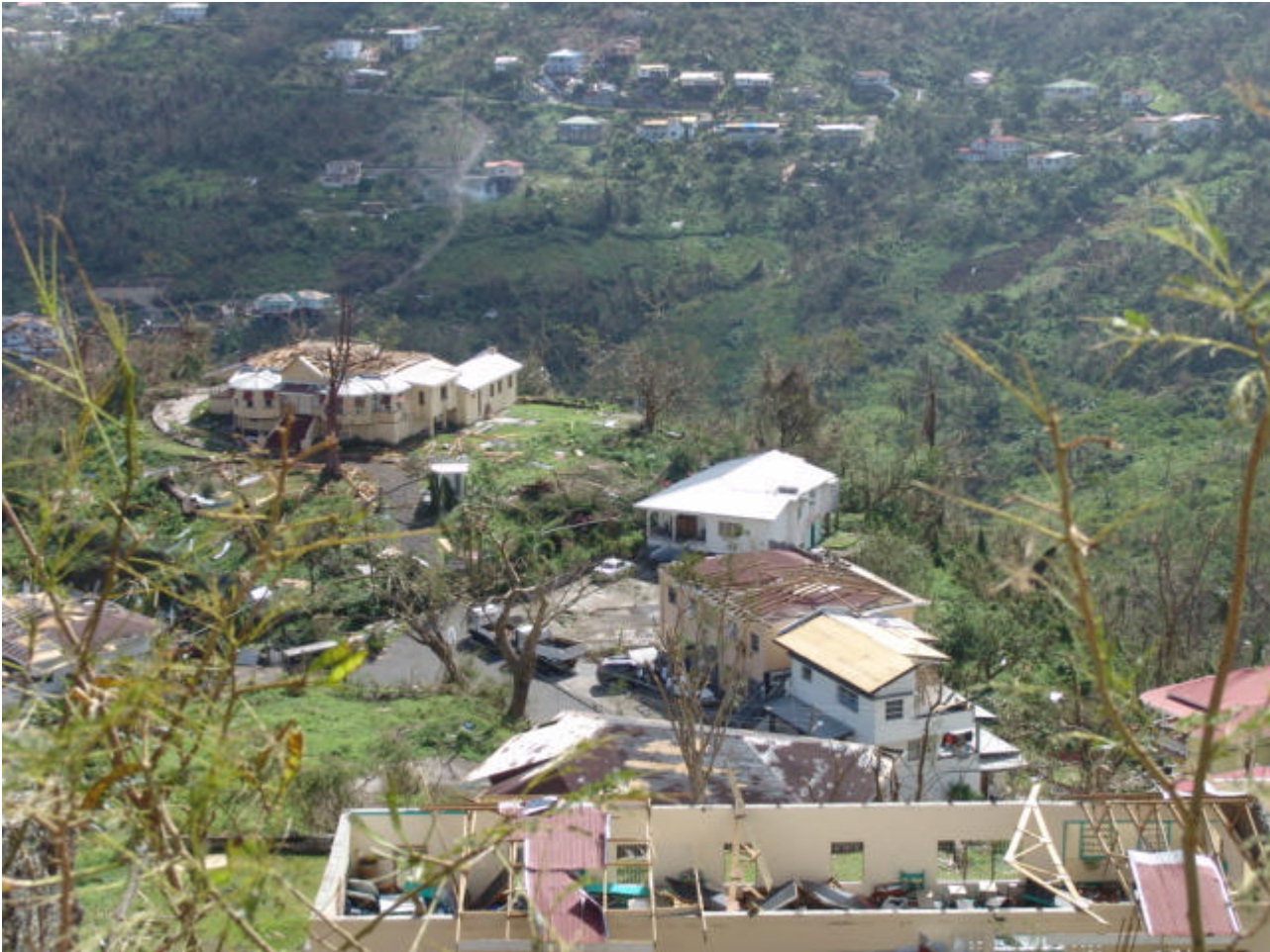
Damaged homes and buildings in Grenada
