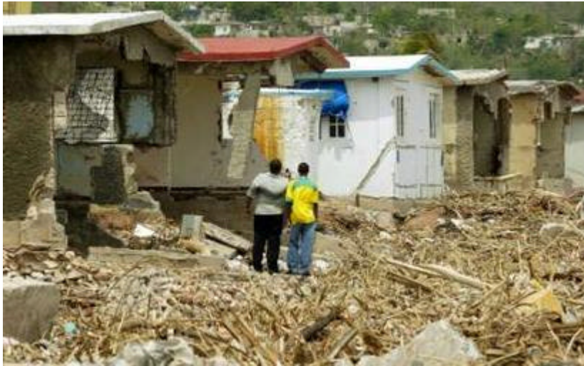
There is major damage to housing in Jamaica following the passage of Hurricane Ivan Photos courtesy of Reuters
