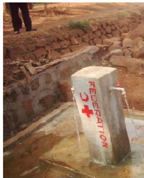
A street fountain constructed with Federation support in Bukavu.
