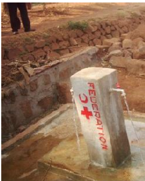
A street fountain constructed by Red Cross in Bukavu.
