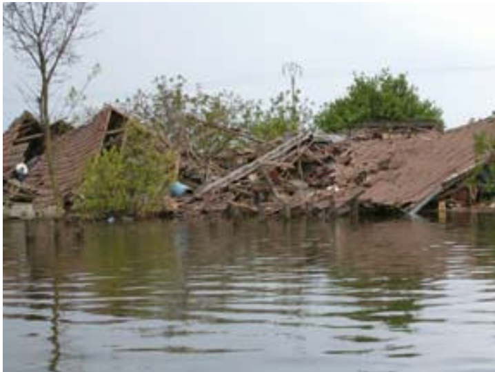
Many houses were devastated in the flooding
