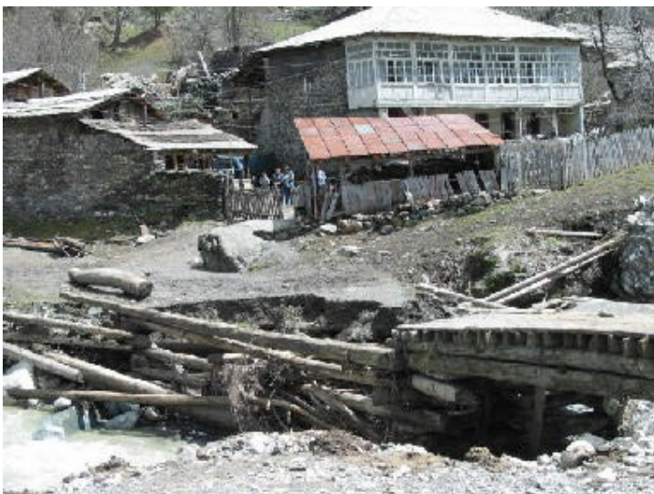
The floods and landslides have caused serious damage to residential buildings and infrastructure
