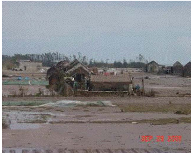
The devastation in the aftermath of Typhoon Damrey. Much agricultural land and property was destroyed.
