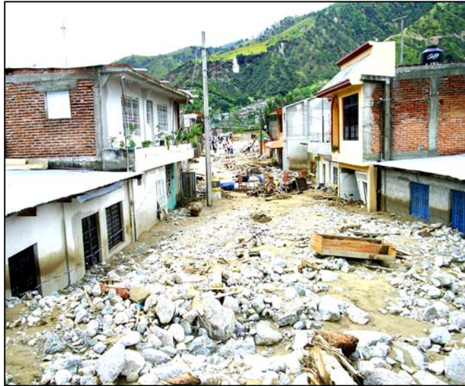
Affected community in Mexico. In addition to destroying houses, floods and mudslides damaged the water system and roads. Source: International Federation.
