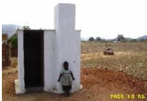
A latrine constructed for a child-headed household in Makoni District, Zimbabwe.
