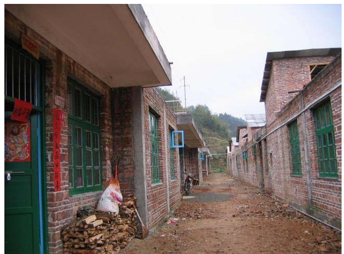
Newly constructed homes in Hunan. International Federation.
