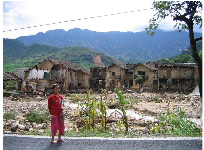
Housing devastation in a flood affected village in Hunan province. RCSC/International Federation.
