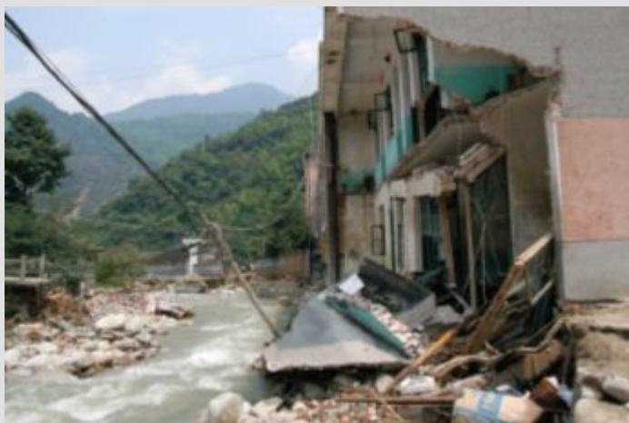
Floods and typhoons wrecked homes and infrastructure.
