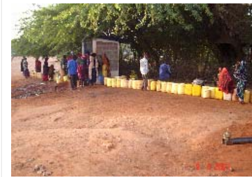
A severe water shortage meant that people queued for many hours in order to draw water from boreholes. This situation was reversed, thanks to pipeline extension and water kiosks constructed by the Red Cross in Mandera.
