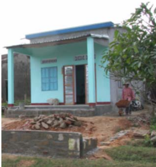
Houses under construction in Hoa Vang District, Da Nang Province.
