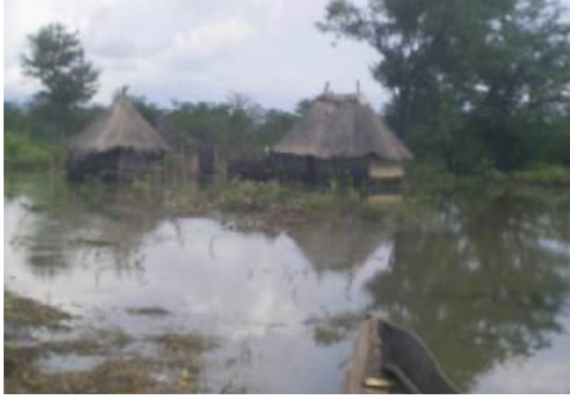
Some of the damaged houses in a rural village in Kazungula district.
