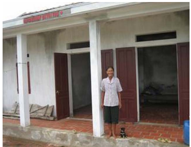
A woman stands in front of a newly built house in Thanh Hoa province.
