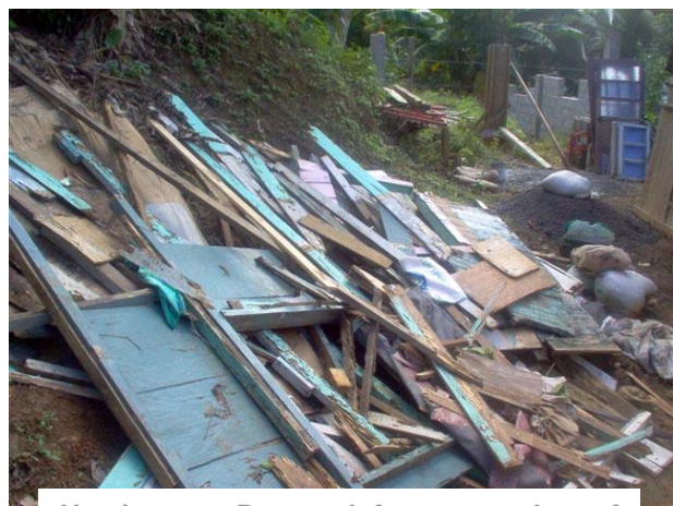
Hurricane Dean left a path of destruction: destroyed house in St. Lucia. Source: International Federation.
