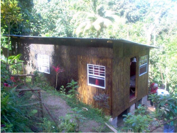
Construction of a new house in St. Lucia. Source: International Federation.
