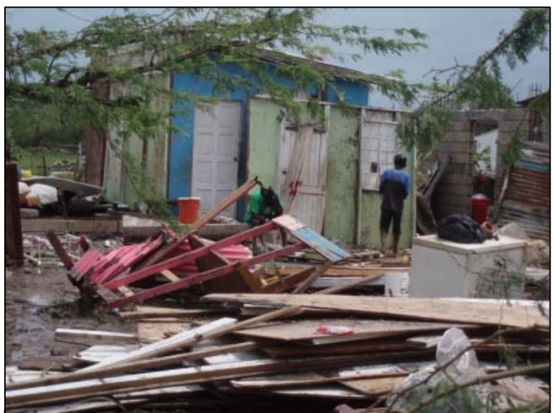
Destroyed houses in Jamaica. Source: Jamaican Red Cross.
