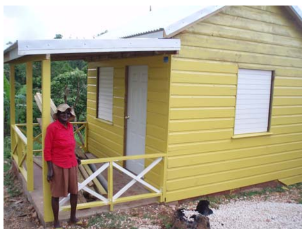
Beneficiary standing in front of her house constructed by the French and Jamaica Red Cross Source: Jamaica Red Cross
