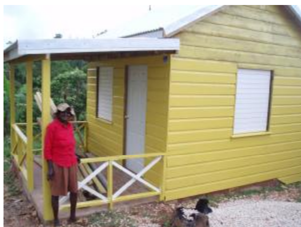
Beneficiary standing in front of her house constructed by the French and Jamaica Red Cross Source: Jamaica Red Cross
