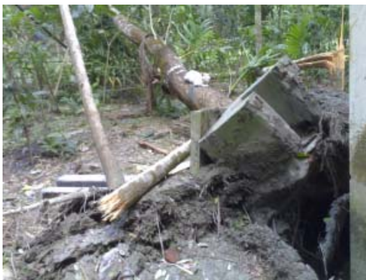
Many latrines were damaged or destroyed by uprooted trees and falling debris, such as this one in Bhola.
