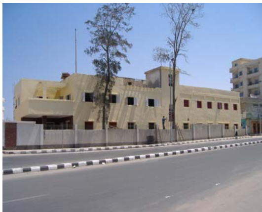
El-Arish warehouse during the renovation
