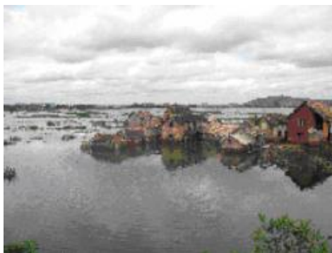
Extensive Flooding following the cyclones.
